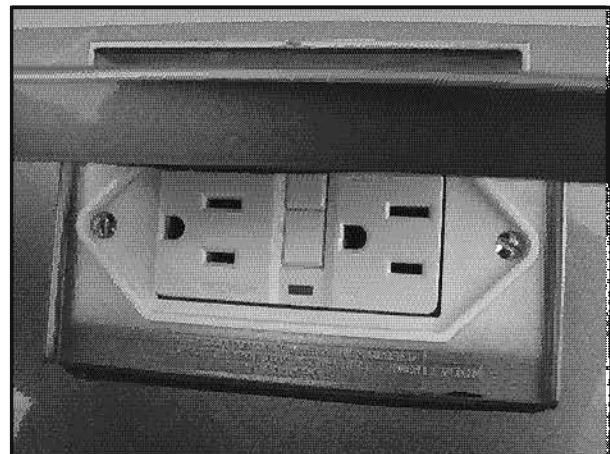
Fig. 6-6 GFCI Outlet (Typical)
